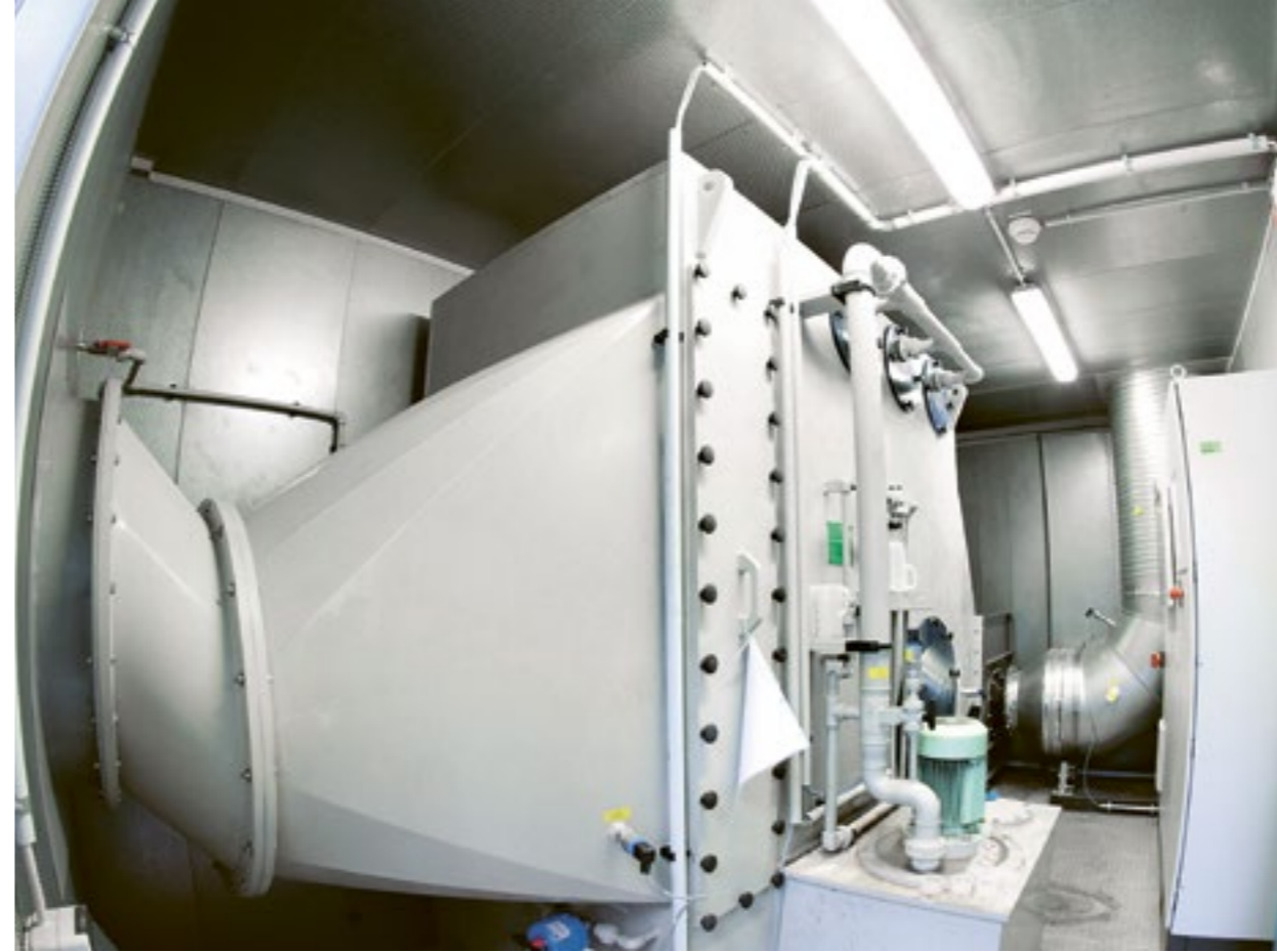
The biological system is alive: To keep it that way, it has to be kept moist.
